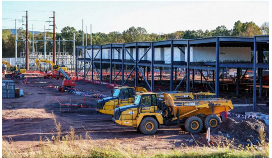
An AI data center building site (Jason Ardan).
